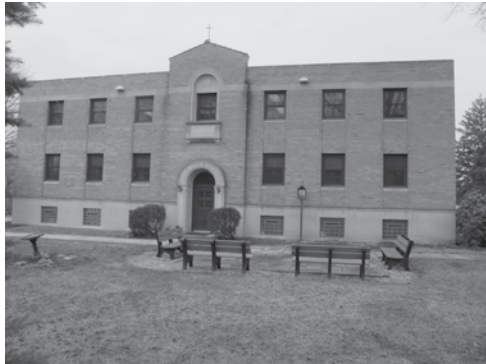
$676,120 Convent & Kindergarten Renovations
