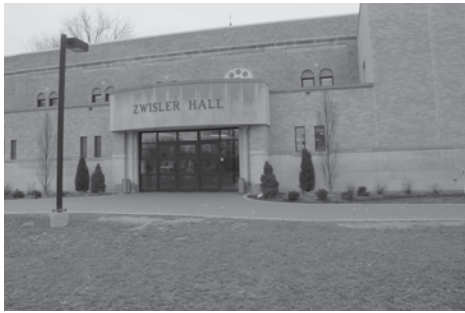
$2,411,779 Zwisler Hall Renovations
