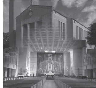
$195,549 Campus Roof Repairs & Replacement
