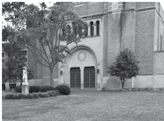
Removed concrete circle drive on Mull Avenue to help with water mitigation
