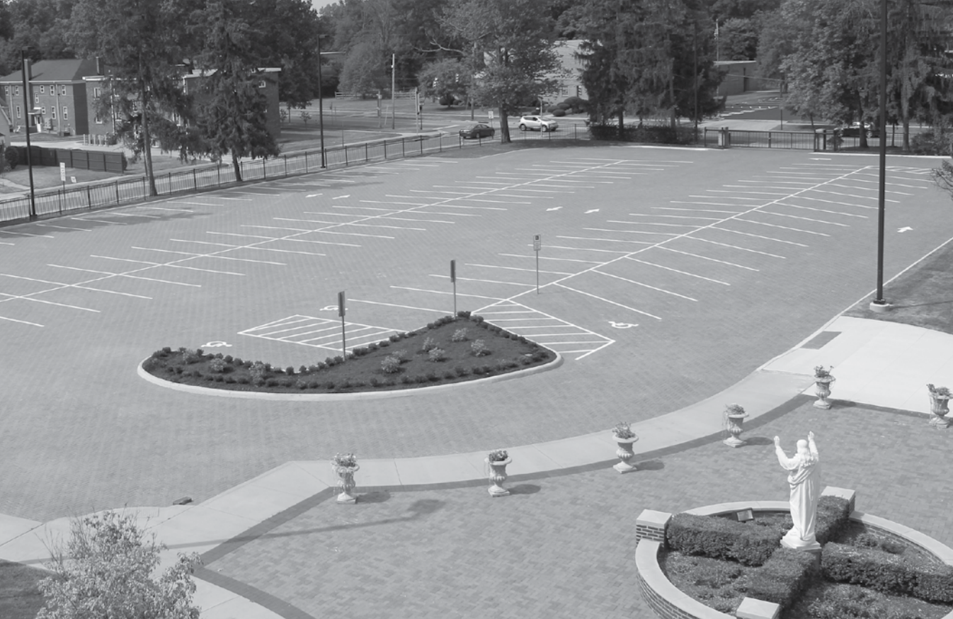
The Completed New Brick Parking Lot! Funded by the generous donors to the Brick Fund and the Rooted in Faith Campaign.
